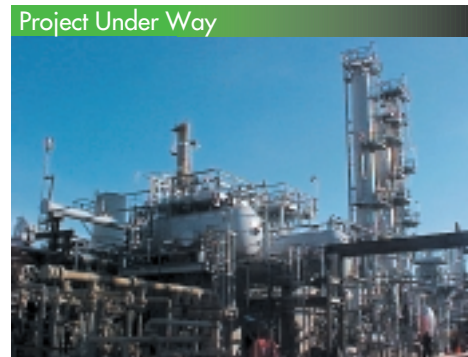
Project Under Way Merox Unit
