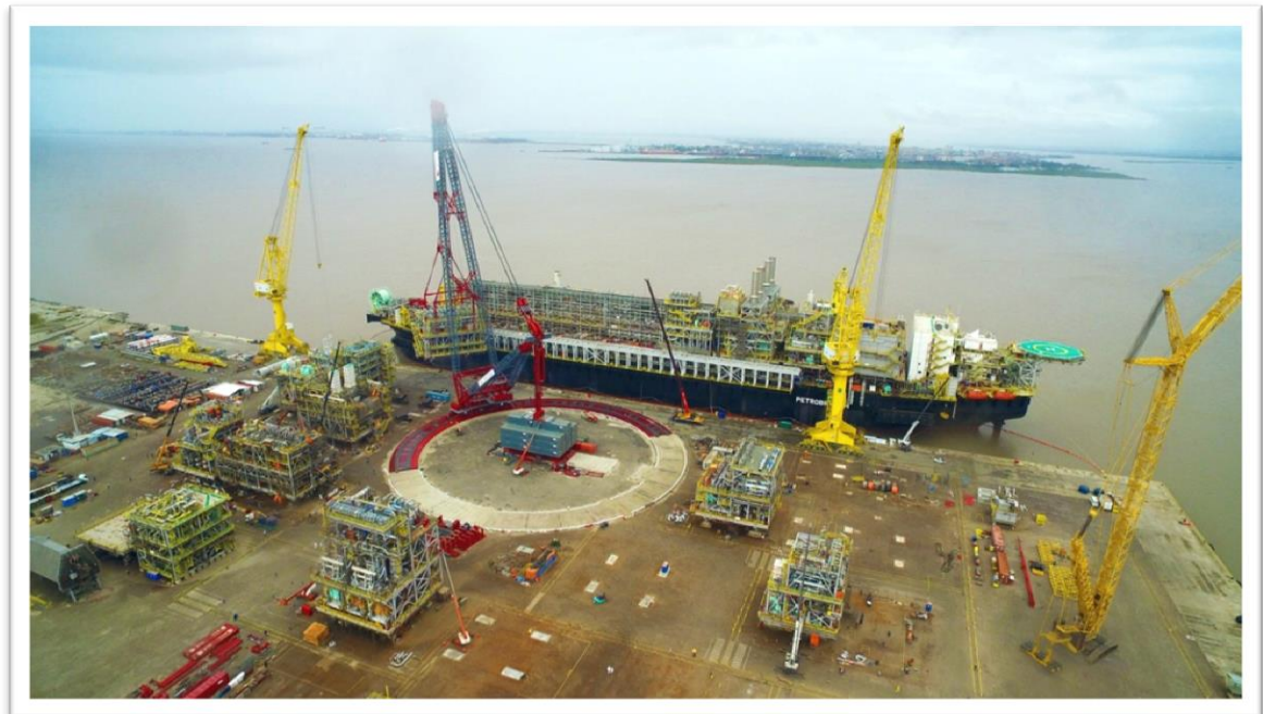
Module installation on FPSO (P-74) (photo: October 2016)
