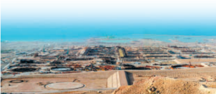
Construction site of South Pars gas processing project, Iran
