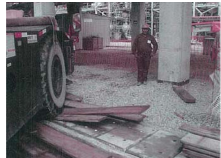
Crane passed over wooden boards
