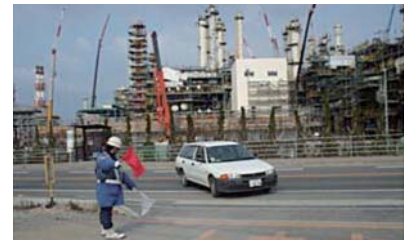
Guard near the site office entrance
