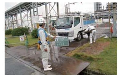
Washing construction vehicle wheels before departure
