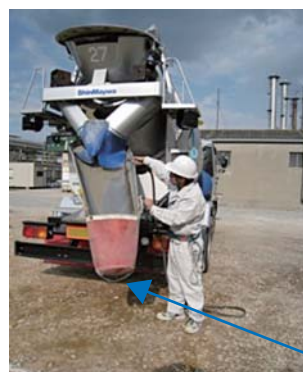
Concrete-mixer-washing water receiving bag
