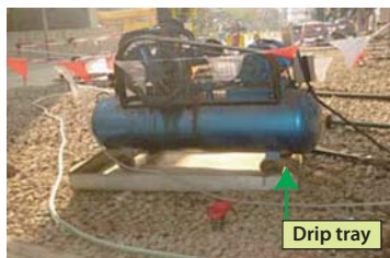
Drip tray for ground contamination control
