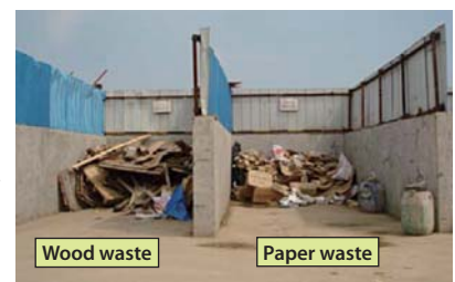
Sorting & storage compartment for construction waste
