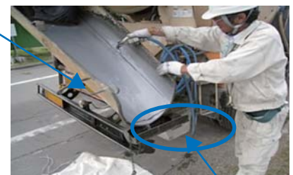
Tank vehicle receiving chute-washing water
