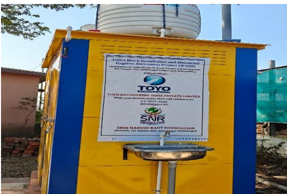
Installation of toilet blocks in 10 tribal schools
