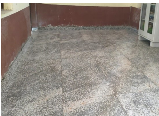
Flooring work of the classrooms
