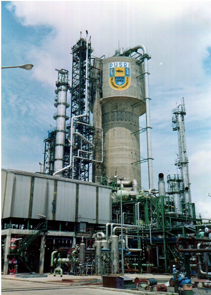
FIG. 8: 1,725 MTPD ACES UREA PLANT FOR P. T. PUPUK SRIWIDJAJA, INDONESIA (PUSRI-1B)
